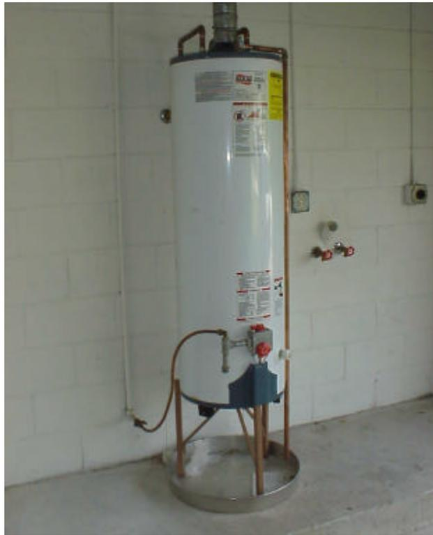
**FIGURE 4: Improper termination of Discharge Pipe**
