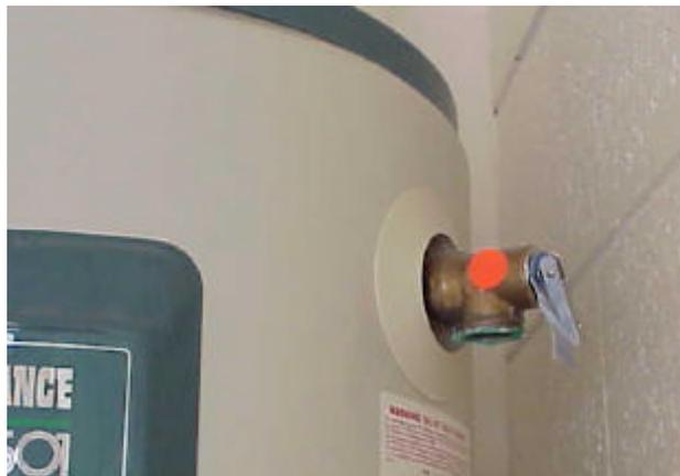
FIGURE 3: Missing TPR Valve Discharge Pipe
