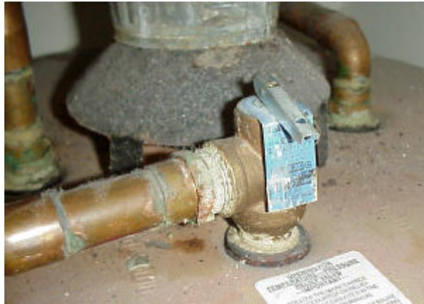
**FIGURE 1: Typical installation of a Temperature/Pressure Relief (TPR) Valve on a Water Heater**
