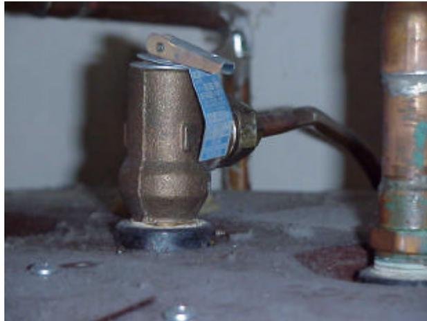
Figure 2: Improperly-sized TPR Valve Discharge Pipe
